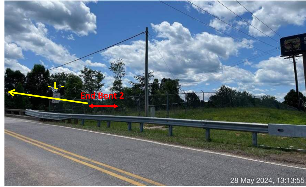
Photograph No. 2: View from north looking at End Bent 2
