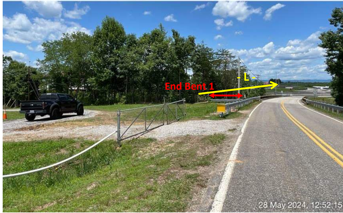
Photograph No. 1: View from south look at End Bent 1
